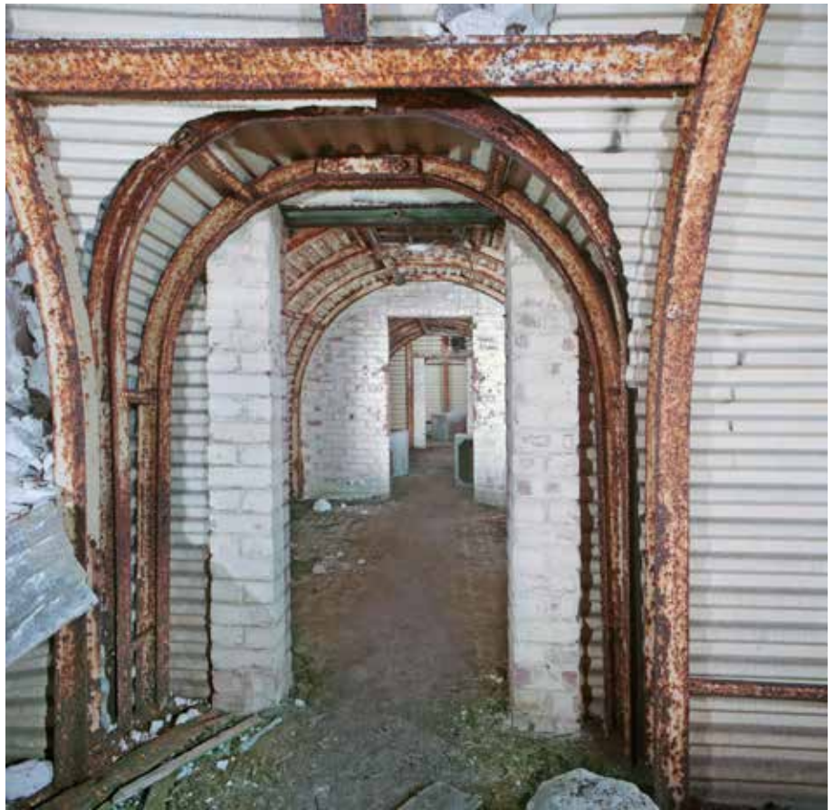
The Emergency hospital and emergency store were located in the cross passage in the Fan Bay shelter. This view is from March 1995. The shelter has always been open and has remained in remarkably good condition considering the access point was a few yards from a public footpath but easily missed if you didn't know it was there. Photo Nick Catford
